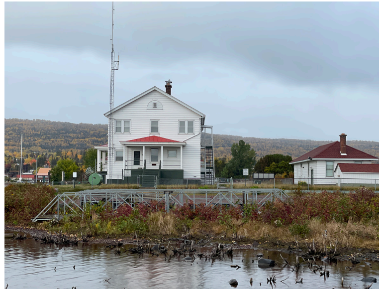
Photo of the existing conditions.
